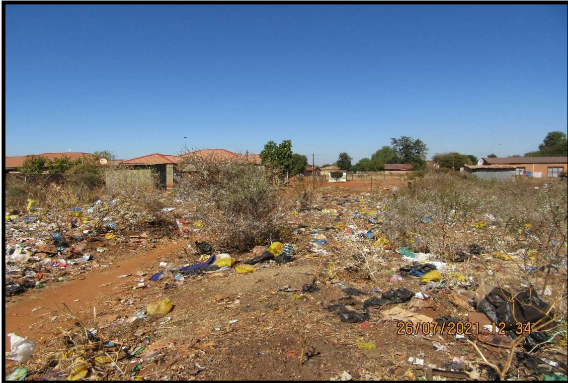
Figure 13: Anthropogenic activities (residential housing and dumping) taking place within 100m of the ARA/BAF powerline
